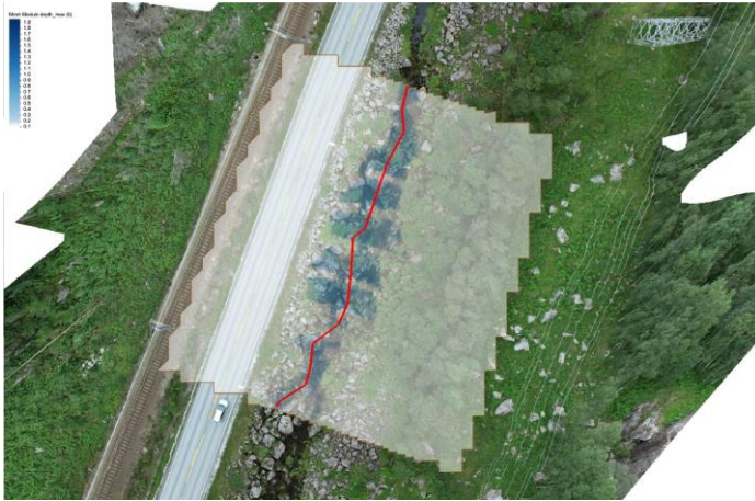
Figure 16: Longitudinal profile through the potential measure in the 2D hydraulic model. The longitudinal profile was chosen to show the water depths and flow velocities over the steps.
